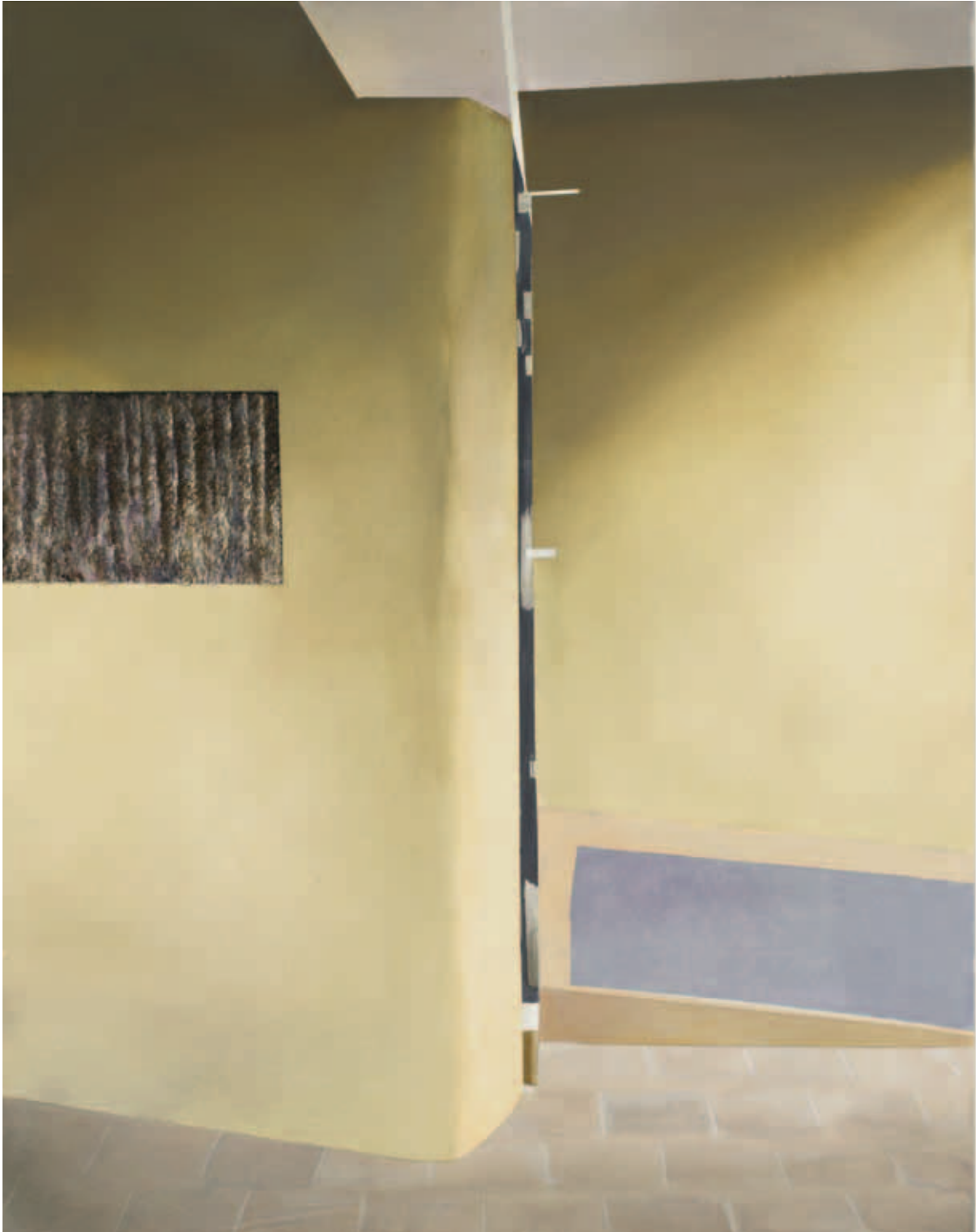
The straw-bale theater of OPEK (Openbaar entropot voor de Kunsten). A «truth window», or an intentional opening in the wall finish reveals the inner straw core.
